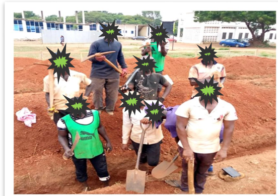
Picture 2- [Initial Foundation Works]
