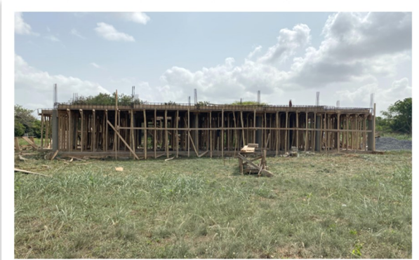
Picture 4- [Decking of the Ground Floor]
